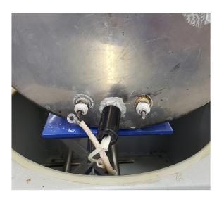
**STEP 5:** Remove all nuts and washers from the new heating element.
