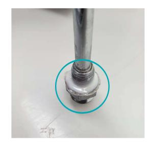
STEP 6: Apply silicone to the nut on one side. This side will face the bath inside base to create a leak proof seal.
