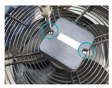
**STEP 7:** Remove the three screws on the terminal from the fan power cord side. Also remove the nut attached to the outside of fan power cord.
