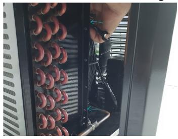
STEP 5: Remove the fan from the chiller housing. BE CAREFUL. WHEN REMOVING THE FAN YOU MAY NEED TO MOVE LINES AND OTHER INTERNALS. BE CAREFUL TO NOT DAMAGE ANY INTERNALS DURING REMOVAL.
